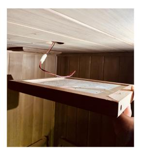
**4.** Fasten the wooden frame of the Chromotherapy Light to the ceiling using the screws supplied. Align the frame centrally above the ceiling hole. Use a tapemeasure to help align the light more accurately.
