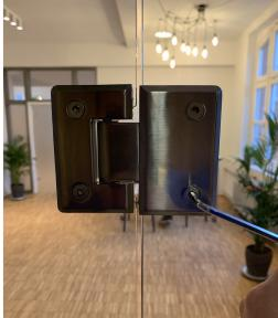
**5.** Also, the part of the hinge which is connected to the glass door should be straight. If this is not the case one of you should go into the sauna and loosen the screws. The other one should lift the door from the outside
