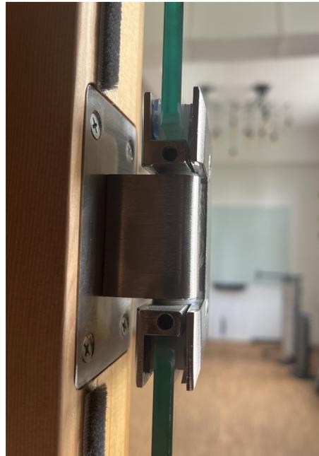
3. Another important part is that the gaps between the glass and the frame should be equal on all sides (including the top and the bottom).
